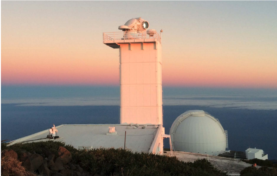
Figure 2.1: The Swedish 1-m Solar Telescope with the distinct white tower at the the Observatorio Roque de los Muchachos on the island of La Palma. The primary imaging element, the 1 m lens which is one of the largest pieces of optical glass in the world, can be seen gazing at the rising sun at the top. Image credit: Rosseland Center for Solar Physics, Oslo.
